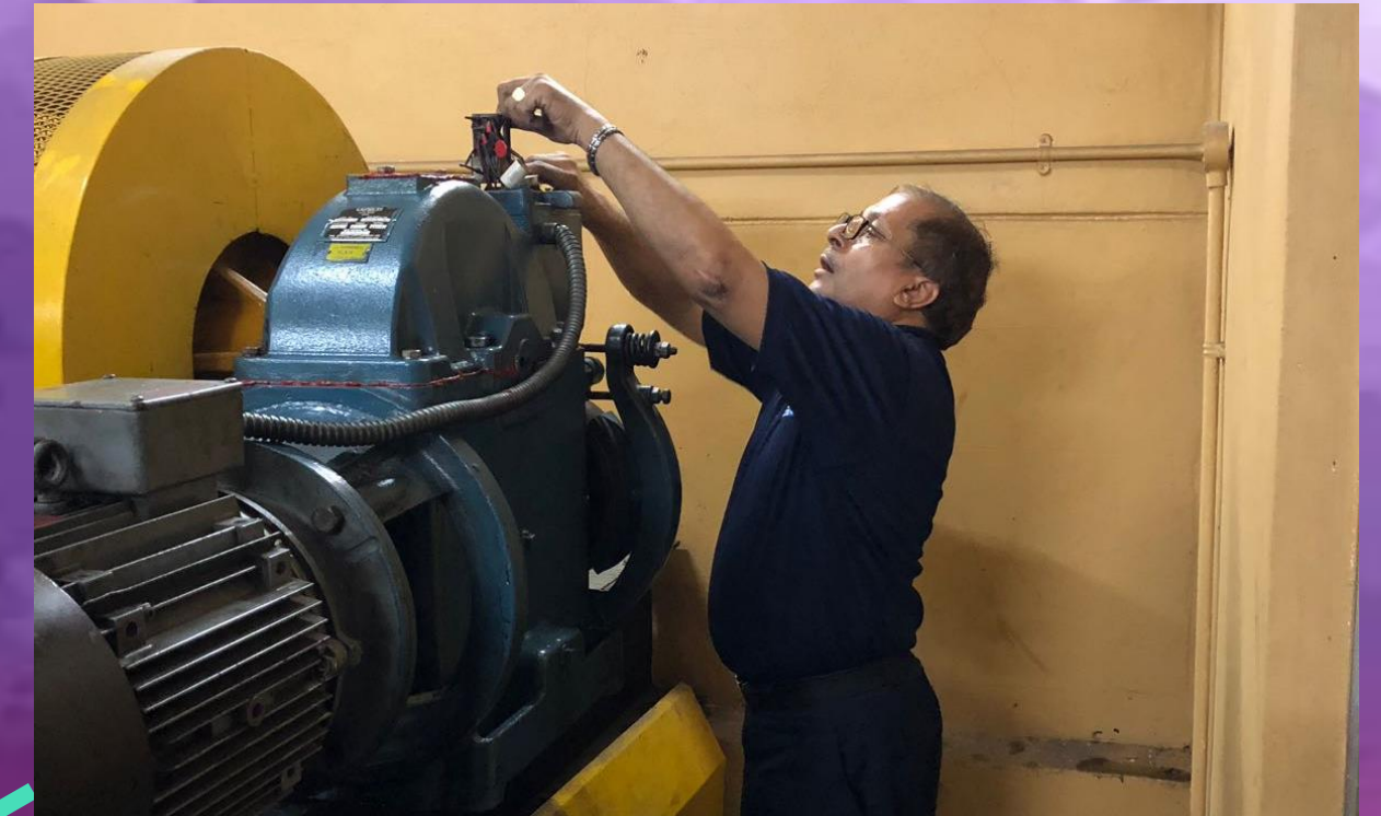
A lift technician conducts lift repair works
