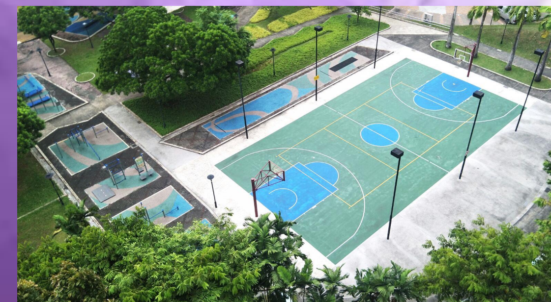
Construction of hardcourt at Mandai Tekong Park Blk 897C Woodlands Drive 50 (Woodgrove)
