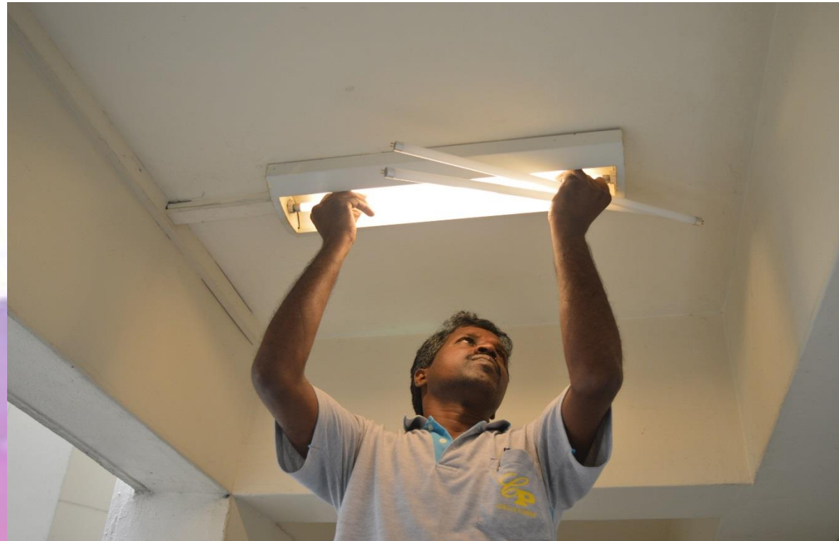
Our electrician replaces a faulty light set
