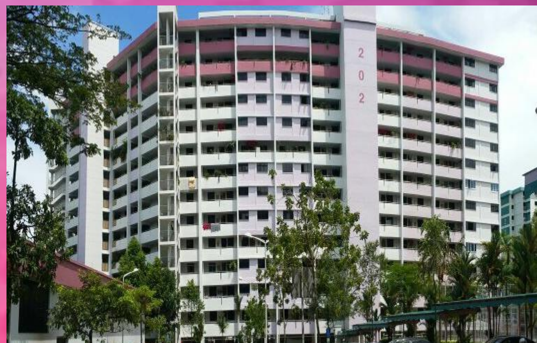
Repainting works completed in February 2017 for Blk 201 to 206 Marsiling Drive (Marsiling)
