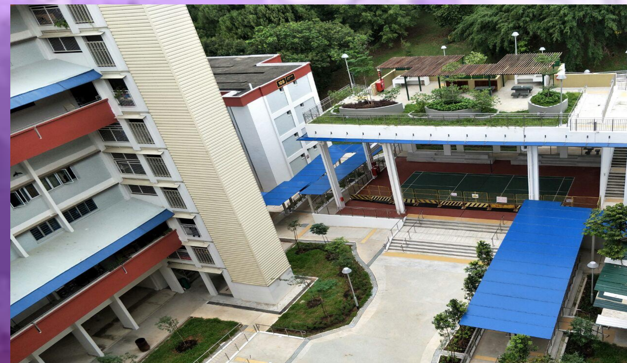
Ongoing construction of Plaza at Blks 113 to 115 Woodlands Street 13 (Woodgrove)
